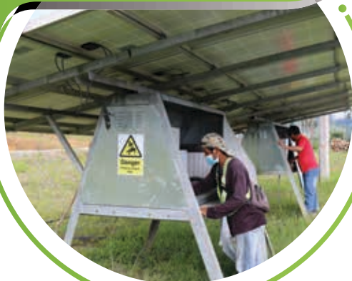
MAINTENANCE DEPARTMENT Routine Maintenance Work of the Solar Panels
